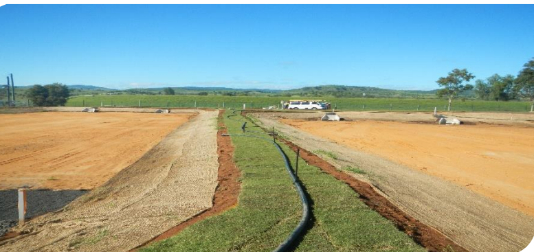
Early construction stage
