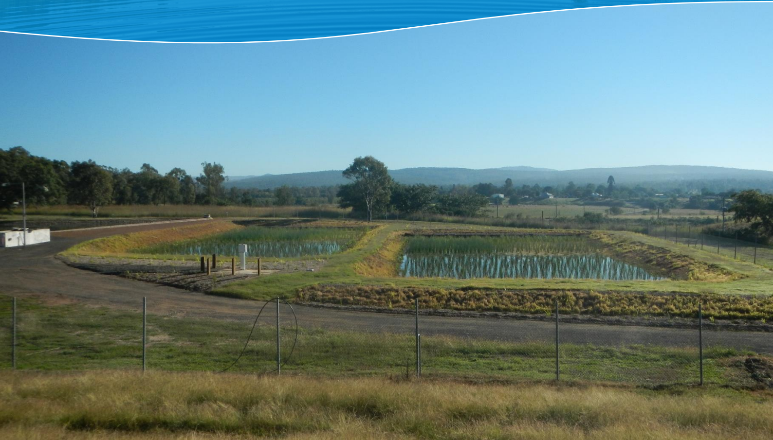
Helidon WWTP- Constructed Wetland
