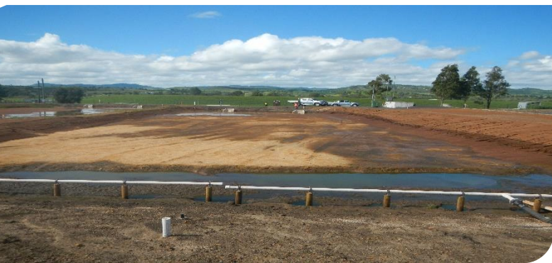
Initial site preparation and wetland construction
